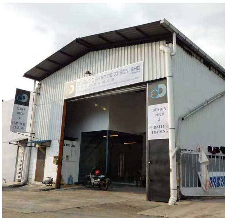
Industrial activities in Taman Bukit Maluri
